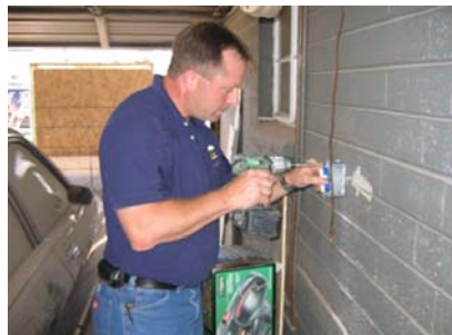
Jason Lacquement of "Super J" Improvements & Repairs.
