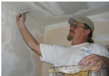
KoKo Stiers of Champion Built Contracting manages the drywall repairs.
